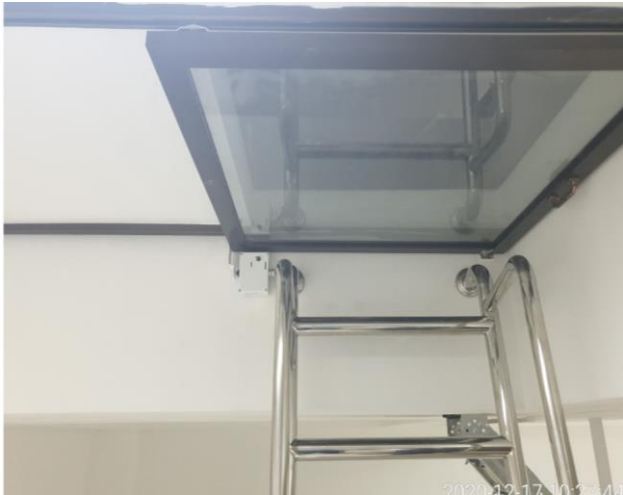
Radome Door Entrance
