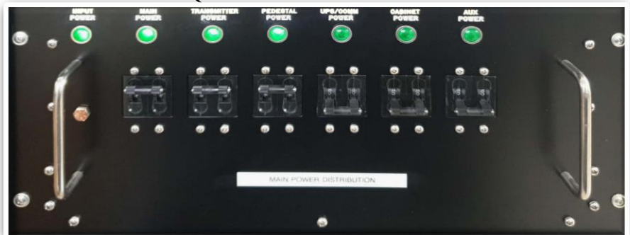
CIRCUIT BREAKER CONTROL PANEL
